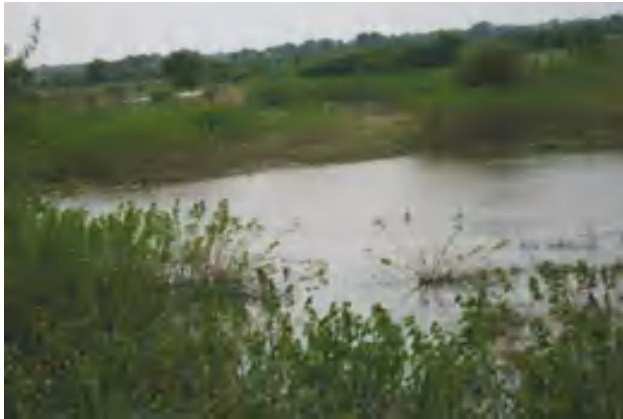
Fig.4.3: Tank with pool of water and weeds growing in it. Moreover, one side of the tank has now even been encroached.
